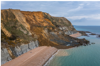
Landslide in Dorset, UK
